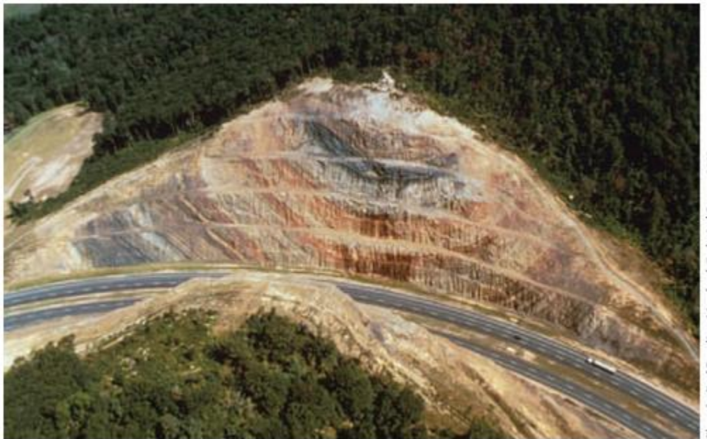
Figure 15. The road cut on sideling Hill, south of the Mason-Dixon line. (Used under the terms and conditions of Rocks and Minerals ( http://www.rocksandminerals.org/Terms-conditions/terms.html ))
