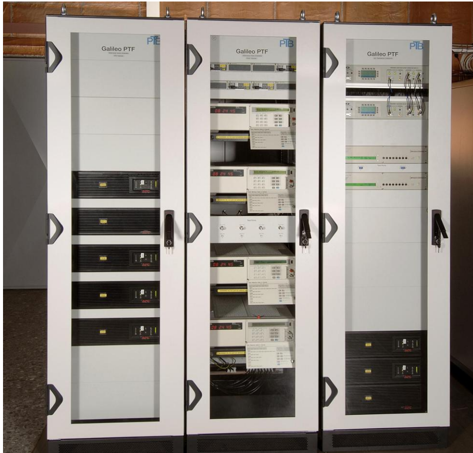
Figure 10. Reference Clock Ensemble (RCE) and GST Realization Subsystem (GRS): The left cabinet contains the uninterruptible power supply, while the Symmetricom 5071A cesium clocks are located in the center cabinet. The cabinet on the right side contains the components of the GRS (see text below for further details on GRS).
