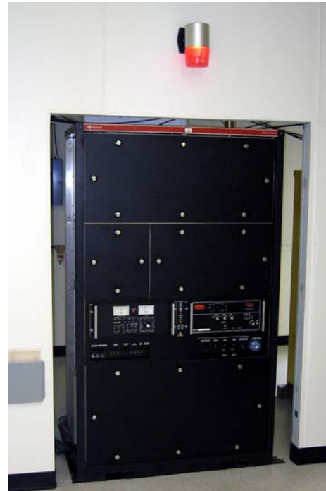
Figure 9. WWV transmitter (FRT-96).
