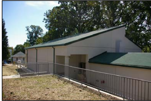
Figure 9. New clock building, November 2006.
