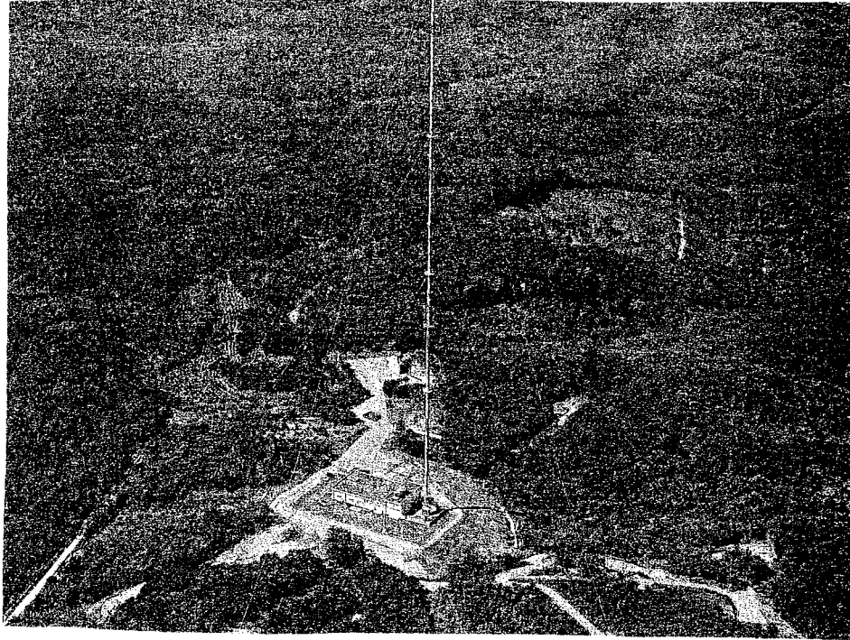
Fig. 2 LF station in Mt. Ohtakadoya
