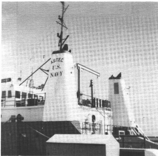
Photo 5 - RV Ranger View of Outside Bridge
