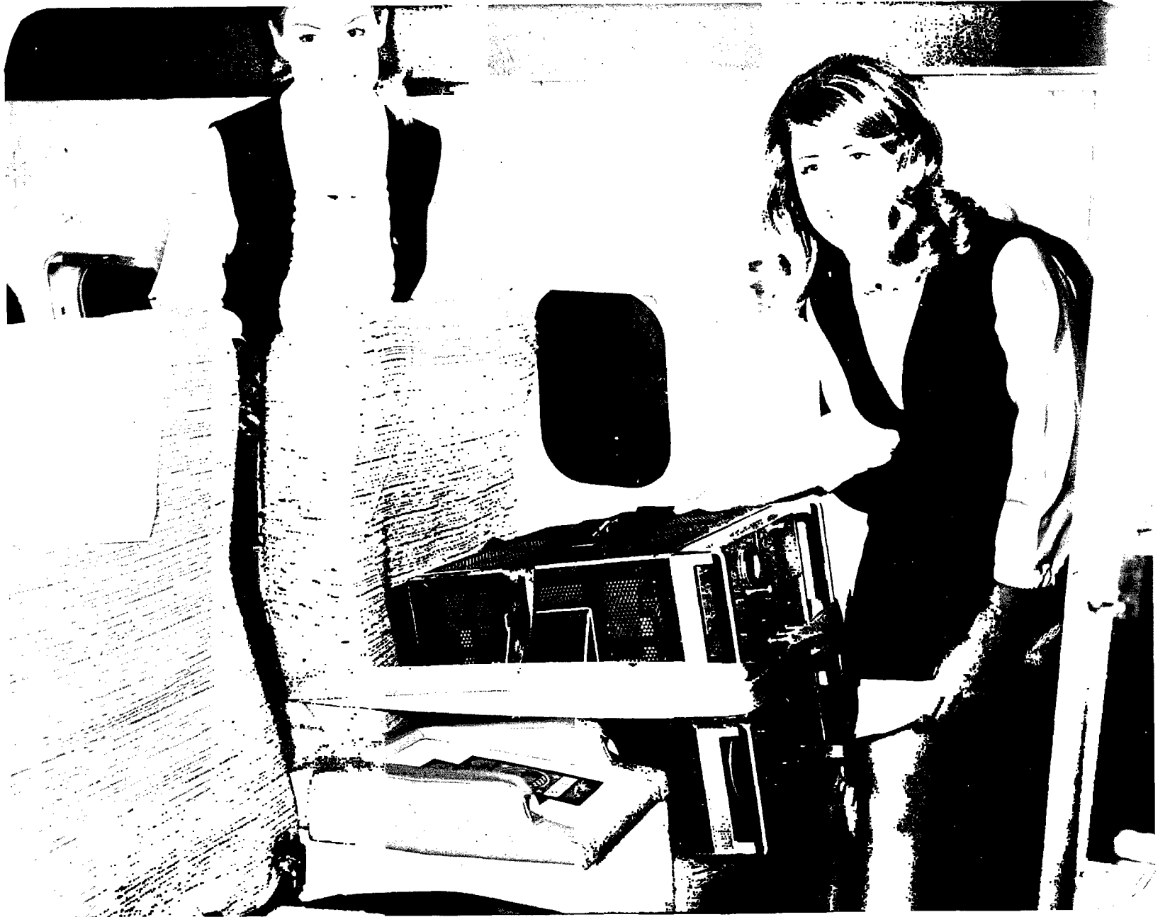
Figure 4. CESIUM CLOCK STRAPPED IN FIRST CLASS AIRLINE COMPARTMENT
