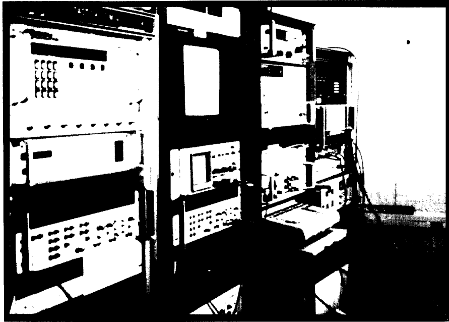
Fig. 2. Earth station equipment.
