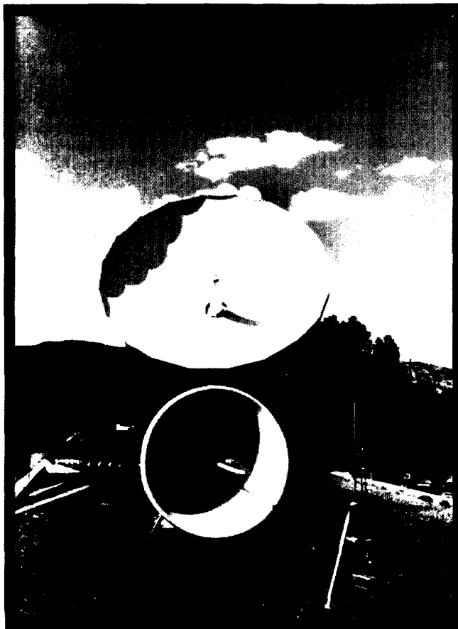
Fig. 1. 6.1 meter antenna used as a hub (shown in background) and 1.8 meter VSAT (shown in foreground).
