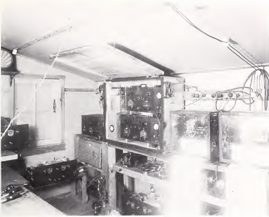
Field-intensity recording equipment in Building No. 3, Kensington, Md. field station. Recorders at right, temperature-controlled receivers at center (note heavy wood housing to stabilize temperature). This equipment was much used in early transmission studies.
