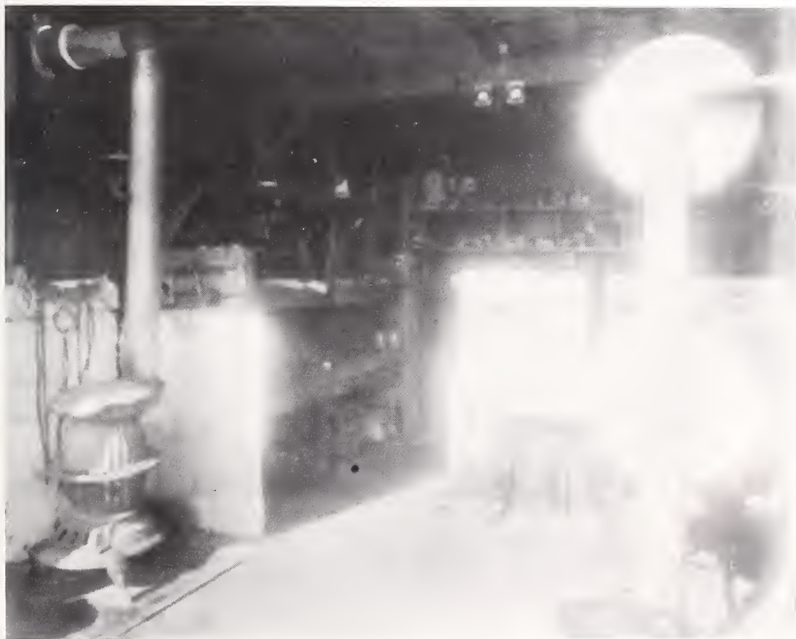
The Radio Section set up its first pulse transmitter (right) for ionosphere measurements in these unpretentious surroundings at its field facility at Potomac Yards (railroad) on the north side of Alexandria, Va., operation beginning July 1930. Previously, dependence was upon a pulse transmitter operated by the Naval Research Laboratory across the Potomac River from Alexandria. At right, can be seen reels for handling the variable length antenna. Reception of signals was at the Kensington, Md. field station, about 20 km distant. By 1932 a pulse transmitter was in operation at Beltsville, Md. and the Potomac Yards station abandoned.
