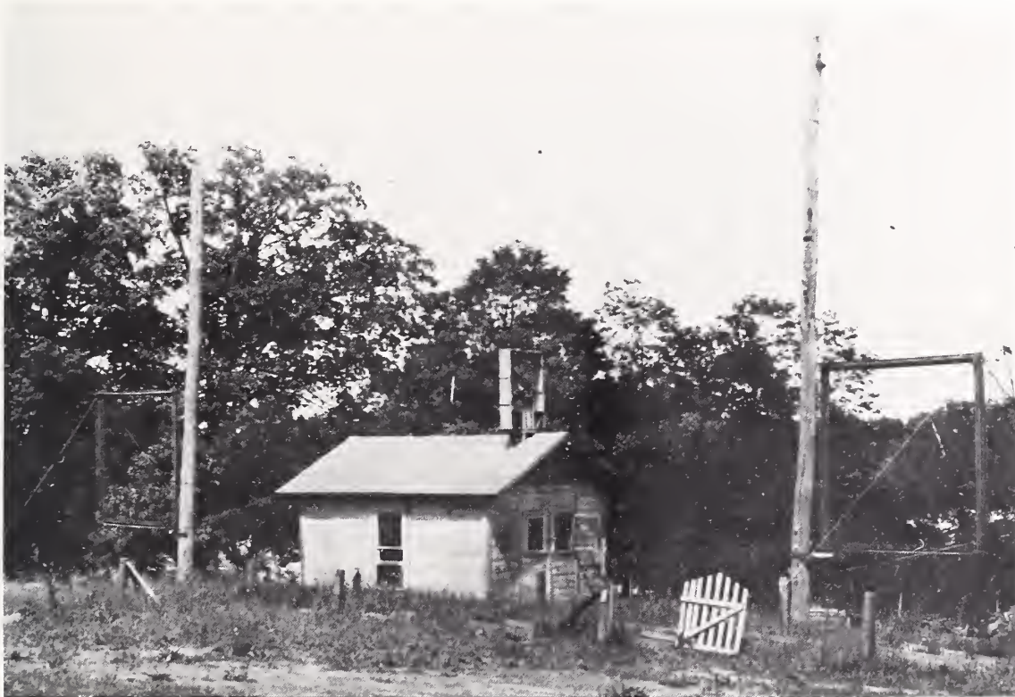
Antenna system of two 10-ft square coils that could be oriented on vertical axes to form a directive crossed-coil radio beacon; located at the "compass house" northeast of Radio Building. This was the original system used by Dunmore in the spring of 1926 to develop an airfield runway localizer for pilot visual indication of course deviation. The transmitter consisted of two RF oscillators, one modulated at 500 Hz, the other at 1000 Hz, each feeding its own coil antenna, but operating at the same radio frequency. Course deviation could be noted by the pilot on a visual indicator controlled by the two modulation frequencies. A receiver located in an open field about 2 miles distance served as the plane's indicator and position in relation to a simulated approach to a radio beacon.
