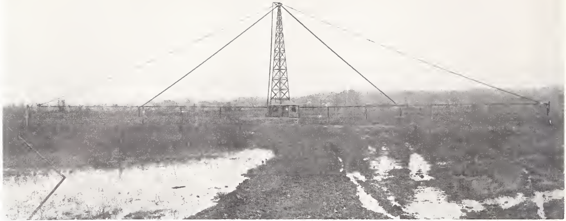
Seventy-foot wood tower radio beacon erected at College Park, Md. Airfield in 1926. Single-wire triangular antennas in two vertical planes replaced the earlier coil antennas used by Dunmore. A goniometer housed at base of tower provided for an equisignal beacon that could be rotated in azimuth for the desired directions. The 4-course beacon was expanded later into a 12-course beacon.
