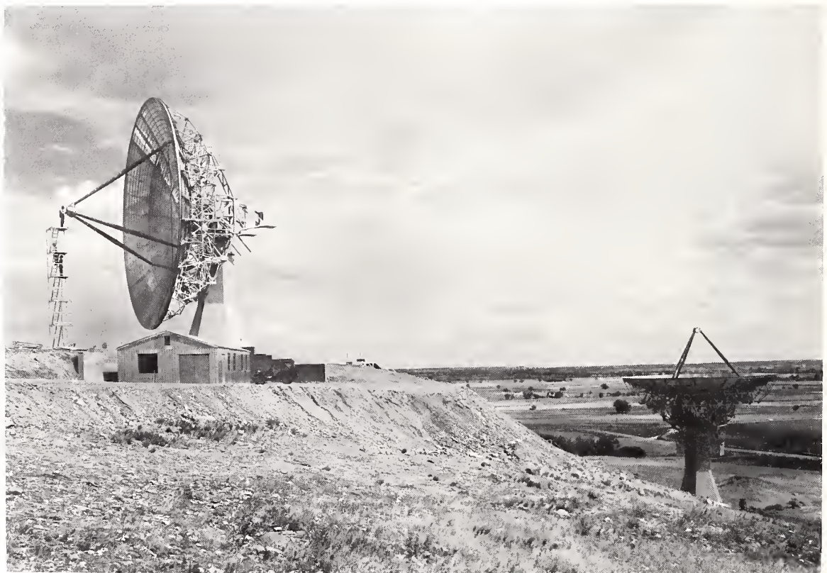
Two 60-foot-diameter parabolic antennas at the NBS Table Mountain field site, north of Boulder. Differences in azimuth and elevation allowed measurement of phase differences (and differences of electrical length) in the arrival of radio waves. The antennas could be moved 90^\circ in elevation between the vertical position (left) and the horizontal (right), and could be rotated 360^\circ in azimuth.
