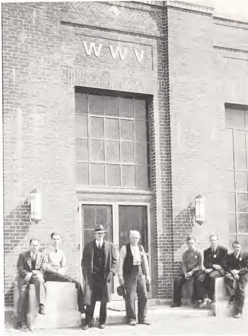
Entrance to station WWV, Beltsville, Md., April 1943, showing operating personnel.
