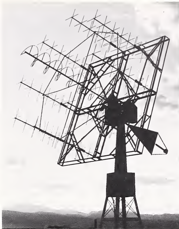
The sun has set behind the foothills to the west of Boulder when this photograph was taken late in the summer of 1964. The steerable antenna was used for tracking Explorer XX (TOPSI sounder) from Gunbarrel Hill. The dual-purpose assembly received signals from the satellite with eight cross-polarized Yagi antennas and transmitted radio commands by the single helix antenna.
