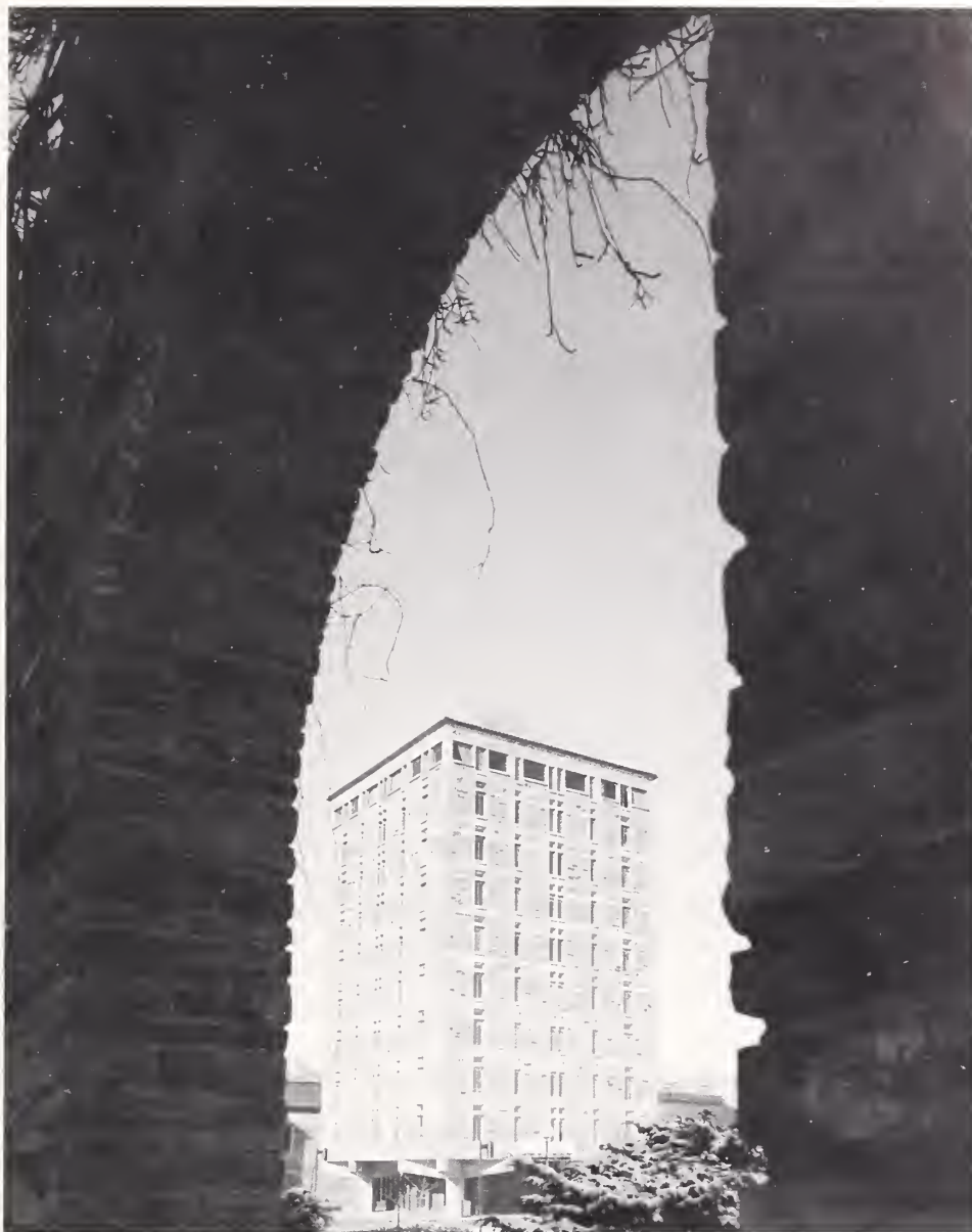
The building of the Joint Institute for Laboratory Astrophysics (JILA) on the campus of the University of Colorado at Boulder. JILA is a joint operation of the National Bureau of Standards and the University of Colorado. The view is looking northeast through an arch of a neighboring campus building.
