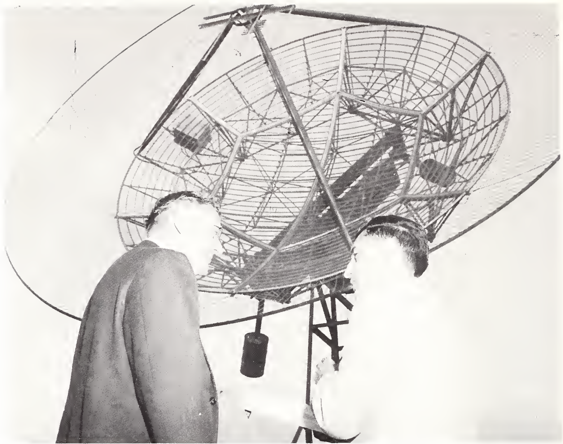
On October 9, 1957, Robert Lawrence (right) of the CRPL informs Gordon Allott, U.S. Senator from Colorado, on the use of a radio telescope for observing Sputnik I. The 40-ft paraboloid reflecting antenna was one of two placed 475 meters apart to form a Ryle radio interferometer. After the launching of Sputnik I on October 4, alterations were quickly made on the equipment to receive the 20- and 40-MHz signals radiated by the Russian satellite. The interferometer was being used to study the perturbations imposed upon radio waves penetrating the ionosphere by observing the emission from radio stars, and particularly from Cygnus A.
