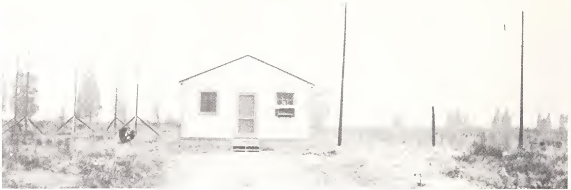
The Warning Service Building was one of four buildings used by the CRPL in its 16-year operation (beginning in 1949) of the Fort Belvoir field station south of Washington, D.C. The antenna structure at left of building was for the direction finder, the antenna at right was for field-intensity measurements of transatlantic circuits.
