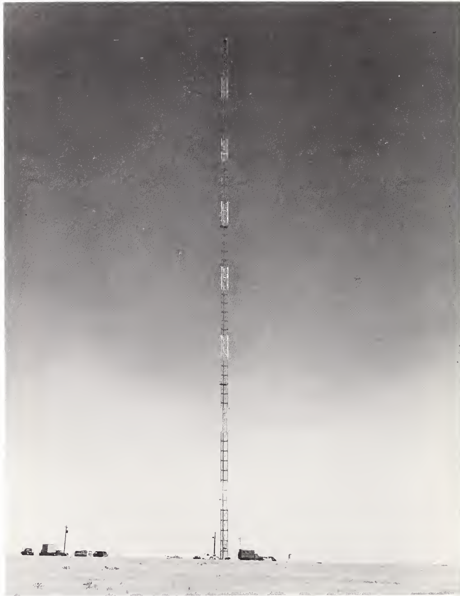
The receiving tower at Haswell, Colo., 96.6 miles (155 km) from Cheyenne Mountain. Provision was made for mounting antennas and meteorological instruments at various levels on the 500-foot tower. The base of the tower is beyond the horizon from the summit transmitter on Cheyenne Mountain; the top is within-the-horizon.
