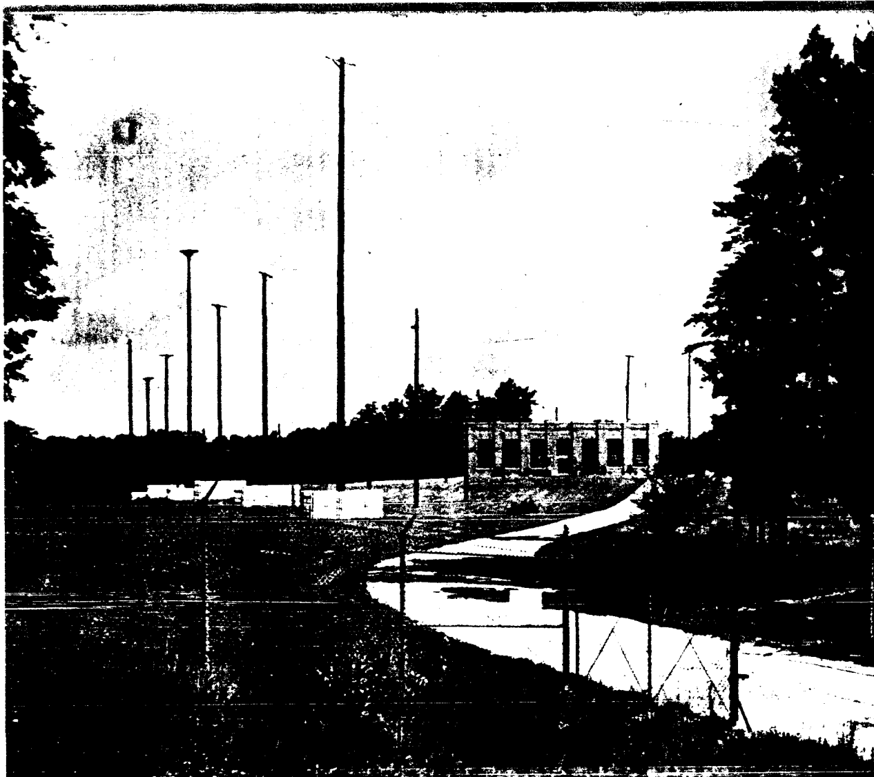
Exterior of tional Bureau ards Radio ing Station W ville, Maryla this station st dio frequenc 5, 10, 15, 20, are transmitt ously, night with accurac parts in 10 Two standard quencies, 600 cycles, are br all radio ca quencies, sta 600 cycles on interrupted o followed by for four min rupted one The telepho support the a tem, from signals are t to all parts of
